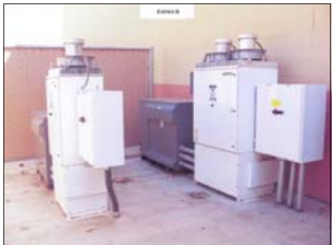
Fire at Mercantile Occupancy, California, April 2009
