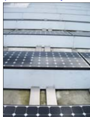
Fire at Educational Occupancy, California, May 2008
