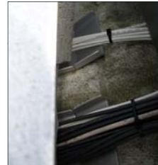
Fire at Educational Occupancy, California, May 2008
