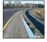
Improved road construction design that included: guard rails to prevent vehicles from striking stationary objects, e.g., bridge abutments, and vehicles from leaving the road, e.g., tight curves, and crossing into on-coming traffic.
